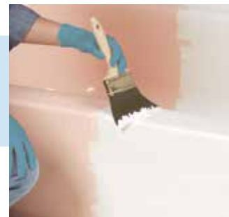
Brush: Apply in THIN, EVEN coats starting at top of surface and working down.
